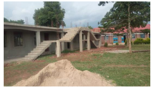
3-Storeyed Building - Stairs added to the building.
