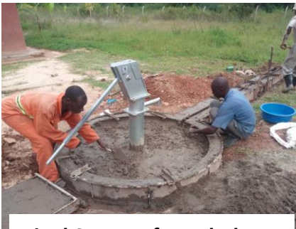
Final Stages of Borehole /Water Well Construction
