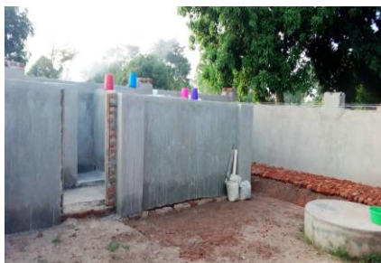
Girls' Bathroom- work goes on
