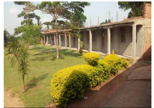
3-storied building - work still goes on
