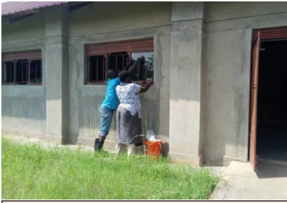
Installing new windowpanes to the dining hall
