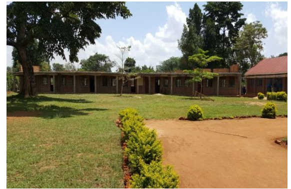
Status of the storeyed building- 2019
