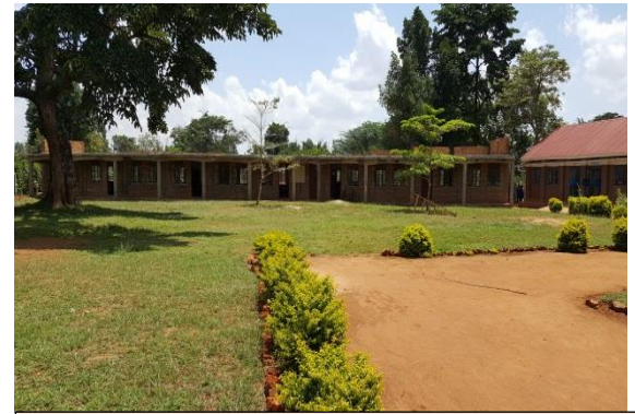
Status of the storeyed building
